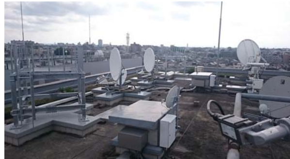
Fig. 9. The rooftop of the NICT building. Two platforms for MWL GT and some TWSTFT antennas are seen.
