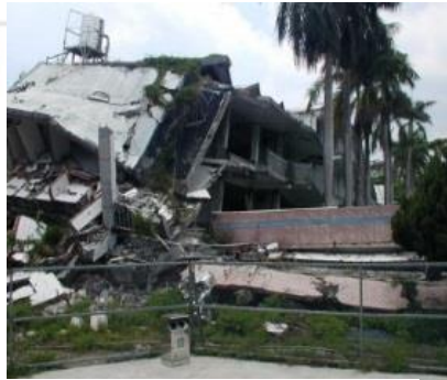
Ji Ji earthquake (1999)
