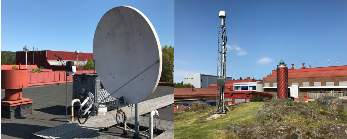
Figure 2: RISE roof-top installation with TWSTFT-antenna and GNSS antennas in the background (picture to left). RISE main GNSS antennas on a concrete pillar and a metal framework construction (picture to right). The main antennas and connected receivers are part of the IGS- and SWEPOS GNSS network. The antenna cables for the main antennas are temperature-stabilized using a water-pipe construction. The main time and frequency GNSS receivers (SP01 and SP02) are connected to the concrete pillar antenna.
