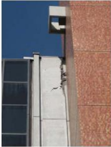
Connecting Hallway between buildings
