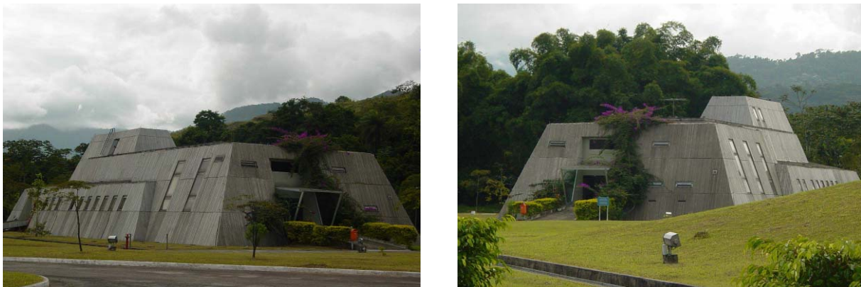
Fig. 1: Building of the Division of Acoustics and Vibration Metrology
