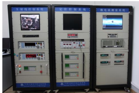
Figure 5. Control, monitor and current measurement system
