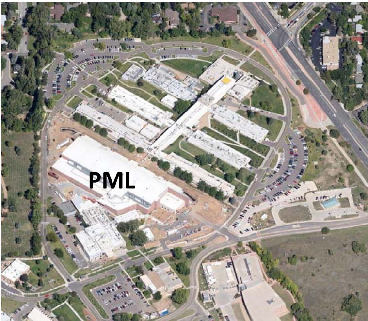
The aerial photo at left shows the new PML (under construction) adjacent to the previous main NIST Boulder laboratory facilities. The older facilities were constructed in 1954.
