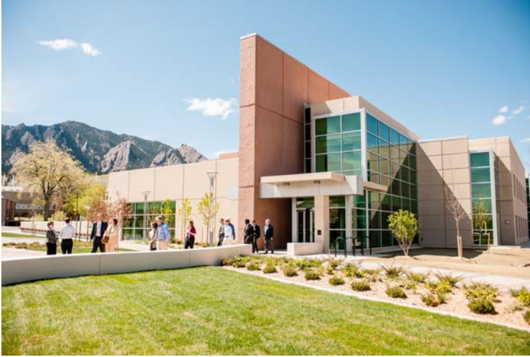
Figure 18. New Precision Measurement Laboratory (PML) at NIST in Boulder, Colorado, USA. The PML provides high performance laboratory space with tight control of temperature, vibration, humidity and air quality to facilitate the most demanding metrology and research. The PML was dedicated in April 2012 and will house many of the NIST Time and Frequency activities.
