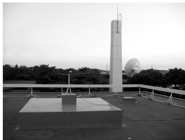
Figure 6. A view of antenna location. The antenna of Timetrace GPS receivers is located on the roof of the main building.
